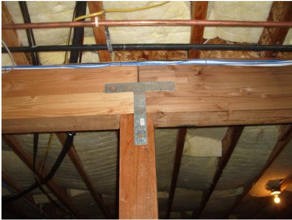
The glu-lam beams and floor trusses in the crawlspace are an upgrade over dimensional lumber. Some framing (“T”) straps are missing, one is shown in the left photo. There is minor wood/soil contact at some of the posts that are bolted to the block walls.
