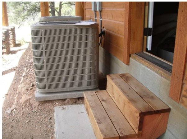
The framing at the decks is above average. Joist hangers are installed, the decks are bolted to the home, and there is flashing at the deck/home. The air conditioner compressors are closer to the home than ideal, and the soil is eroding from under the concrete pads under the compressors. There is a high step at the wood steps into the crawlspace.
