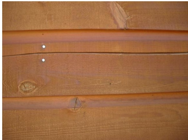
There are gaps and split boards at the wood siding.
