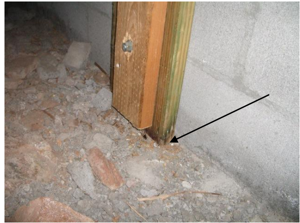
The glu-lam beams and floor trusses in the crawlspace are an upgrade over dimensional lumber. Some framing (“T”) straps are missing, one is shown in the left photo. There is minor wood/soil contact at some of the posts that are bolted to the block walls.
