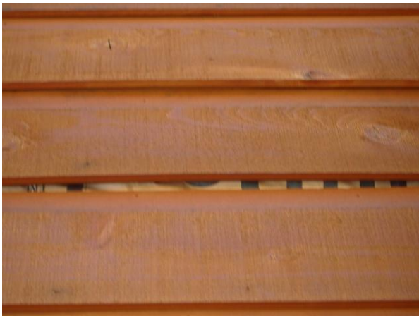
There are gaps and split boards at the wood siding.
